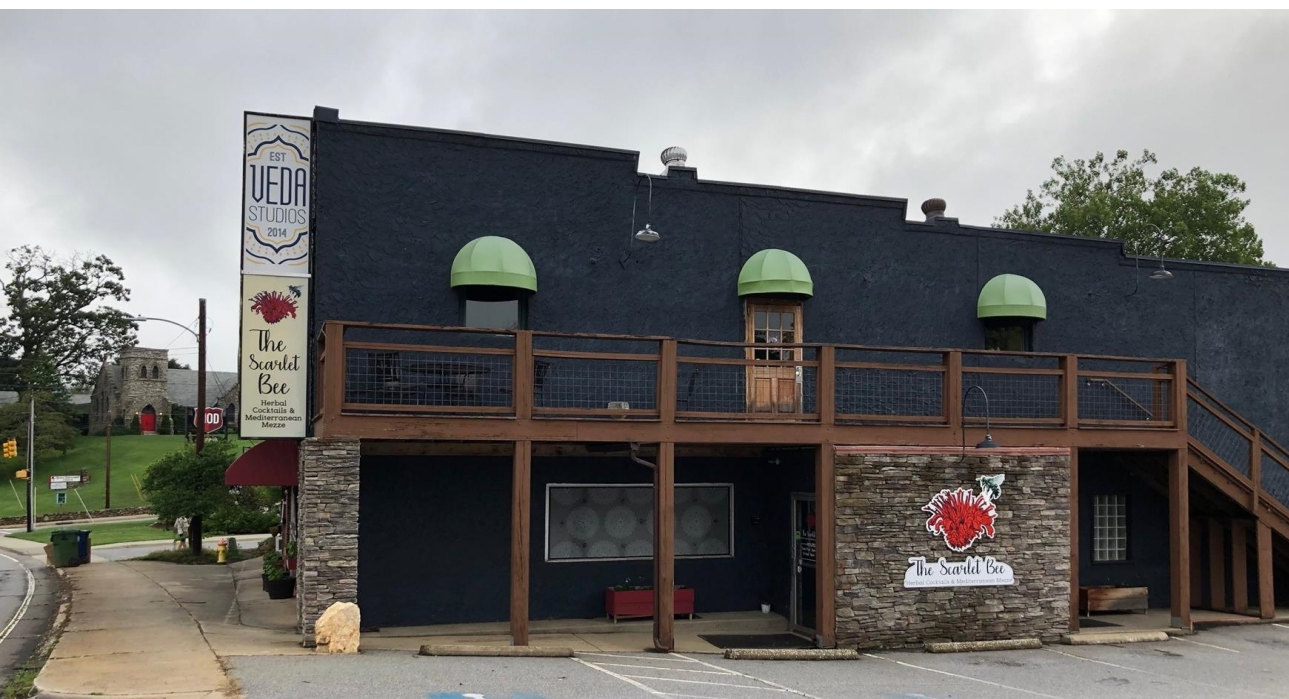
Side view - south looking north
