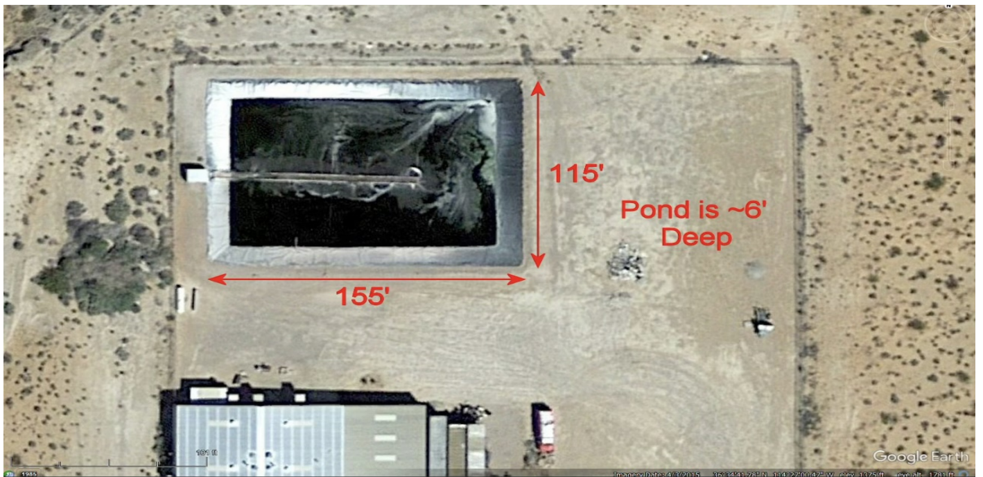
Overhead view of the double lined HDPE evaporation pond and surrounding containment area.
