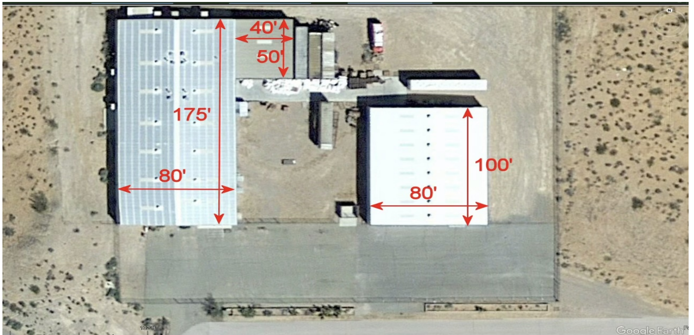
Overhead view of building improvements and paved yard area.
