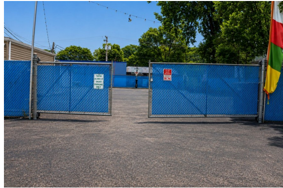
Secured, gated lot
