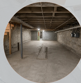
ADDITIONAL BASEMENT STORAGE
