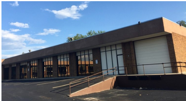
OVERHEAD DOOR BAY
