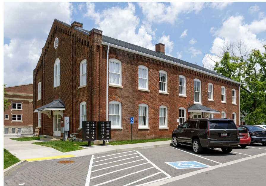
BUILDING D / 6,443 SF
