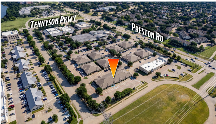
Aerial — Preston Rd & Tennyson Pkwy
