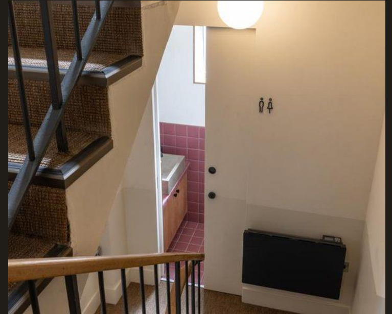
Refurbished Common Parts
