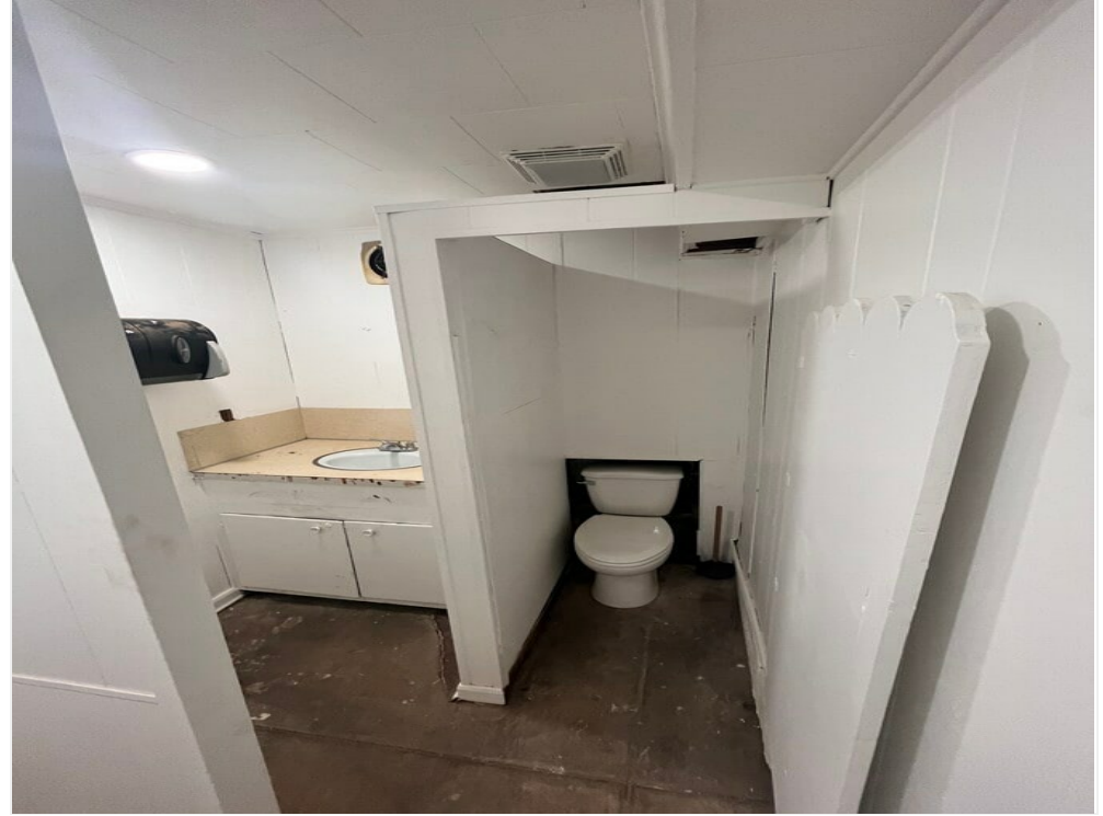
View of Warehouse Bathroom
