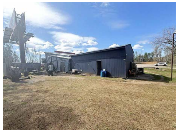
East Side of Building
