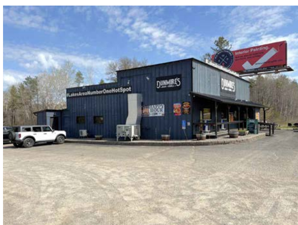
West Side of Building
