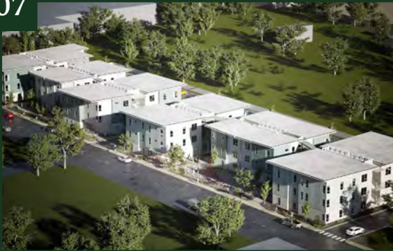
Lemen Avenue Affordable Housing 1224-1230 Lemen Avenue | 73 Units
