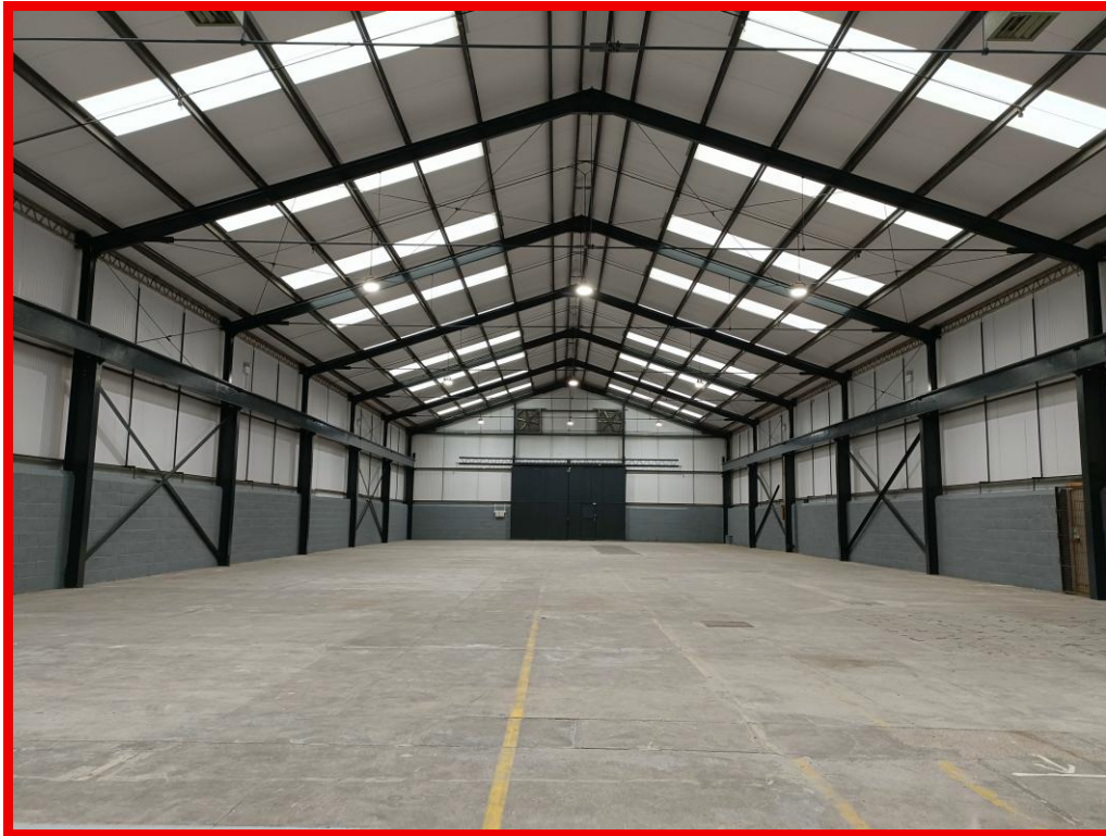
View of warehouse
