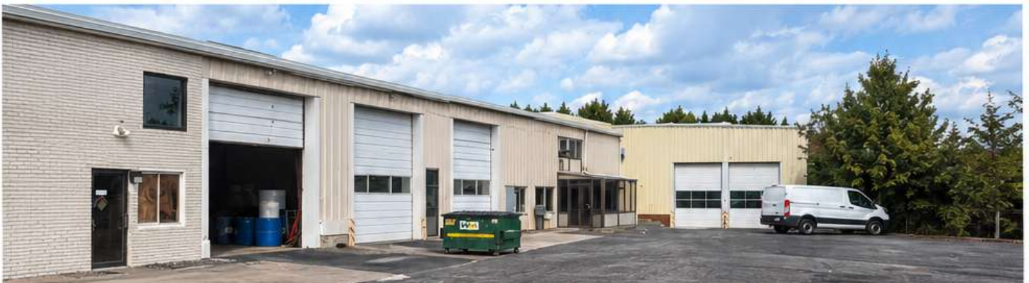
SIDE WAREHOUSE – 3 DRIVE-IN DOORS
