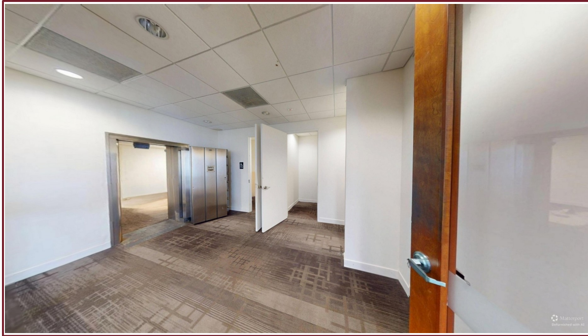
Former bank vault access
