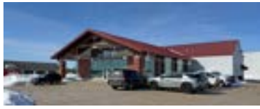
6.) Standard Electric - Branch 22 1100 Gornick Ave, Gaylord, MI Size: 10,000 SF | Built: 1980
