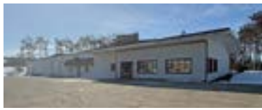
12.) Standard Electric - Branch 5 1815 Dickerson Rd, Gaylord, MI Size: 11,918 SF | Built: 2000
