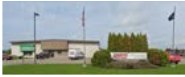
7.) Standard Electric - Branch 18 2640 Davitt St, Sault Ste Marie, MI Size: 11,122 SF | Built: 1985
