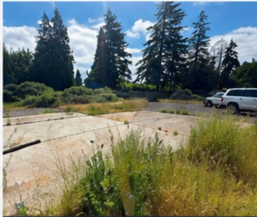
Existing utility and slab area
