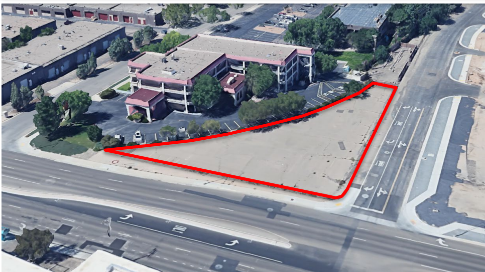
SITE AERIAL - YALE BLVD SE
