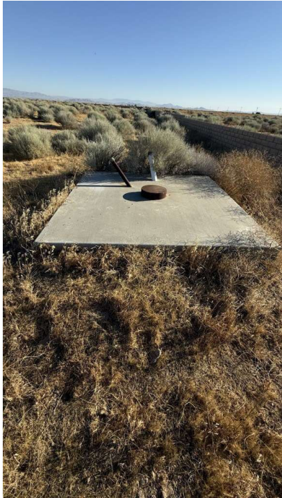
Second onsite well, capped at the surface — discovered during recent well work, June 2026.
