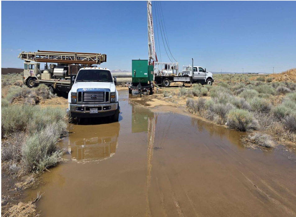
Independent Well Drilling rig and support equipment on site, June 2026.
