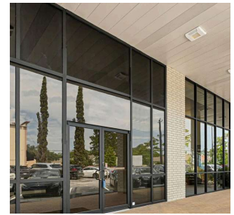
Suite F — Storefront & Glass Facade
