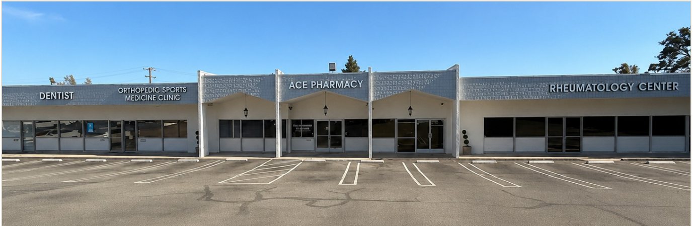
BUILDING ELEVATION — ±9,464 SF MULTI-TENANT MEDICAL / PROFESSIONAL BUILDING AS VIEWED FROM THE W. FOOTHILL BLVD. PARKING FIELD. TENANCY INCLUDES DENTAL, ORTHOPEDIC SPORTS MEDICINE, PHARMACY AND RHEUMATOLOGY USERS.
