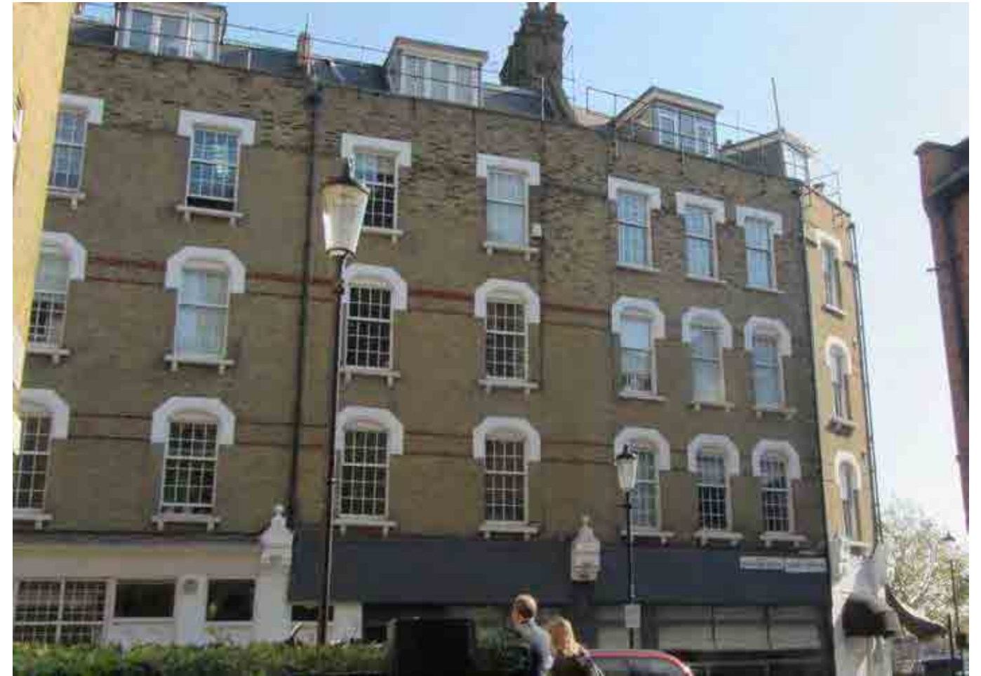
1. Elevation to Riley Street
