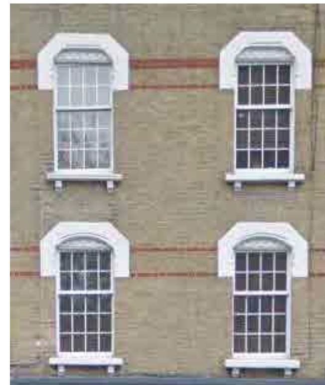
Traditional materials of the main facade
