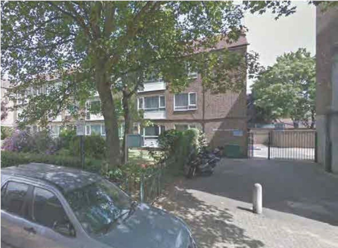
3. View towards Cremorne Estate
