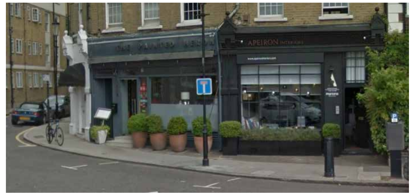
3. Existing Shop fronts
