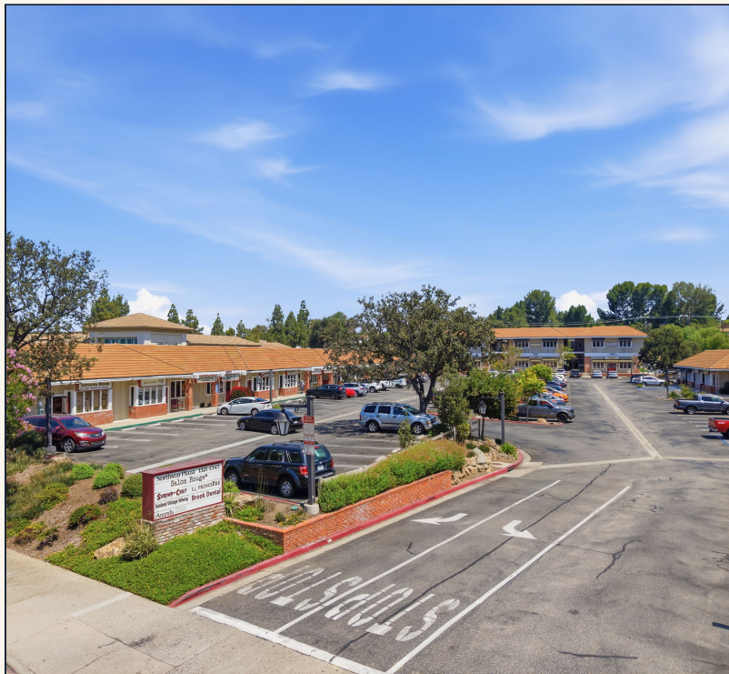
Aerial — four-building plaza with central parking court
