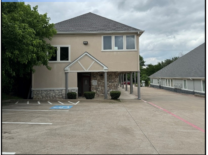
Back of Building
