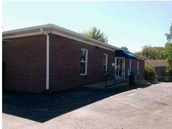
Front View of Building
