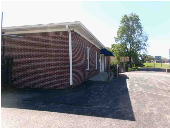
Front View of Building
