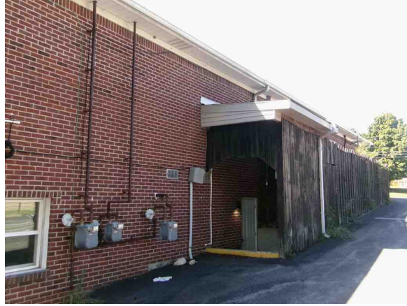
East Side of Building
