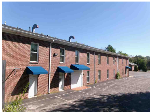
West Side of Building
