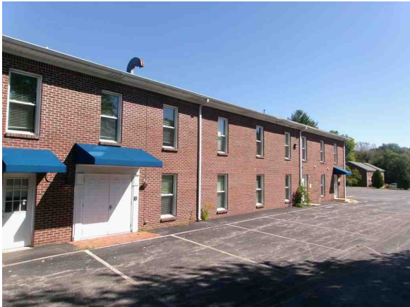
West Side of Building
