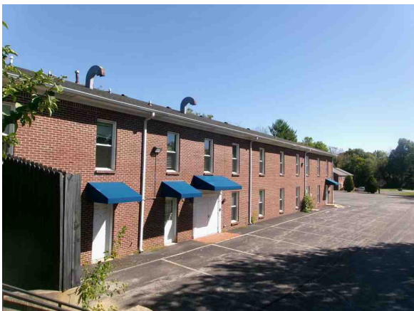
West Side of Building
