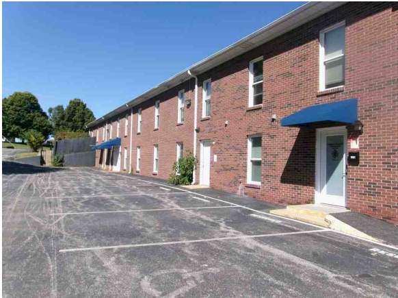
West Side of Building
