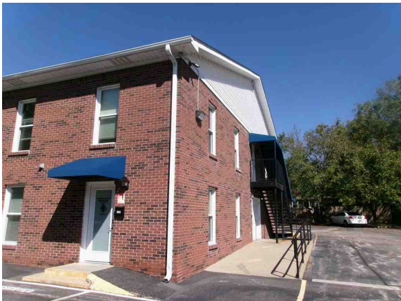
Rear of Building
