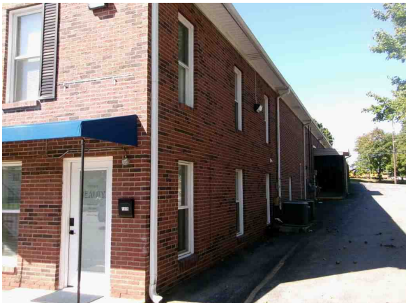
Rear of Building
