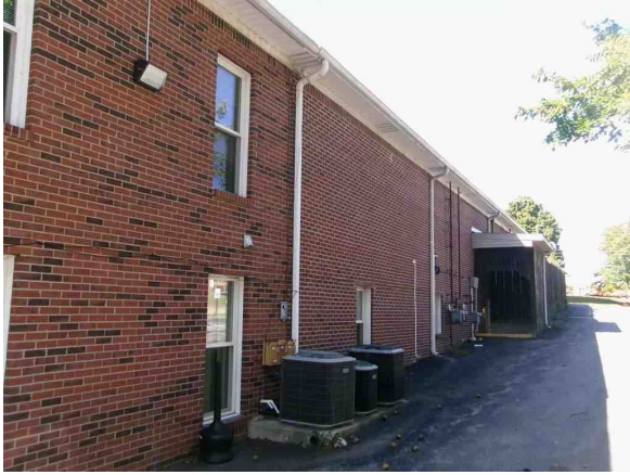
East Side of Building
