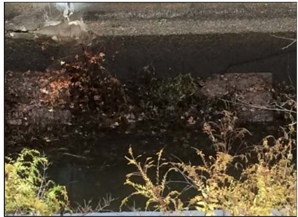
Photo 10: Close-up of canal wall showing presumed concrete patch of penstock #1 which once fed tailrace #1 (11/19/15).
