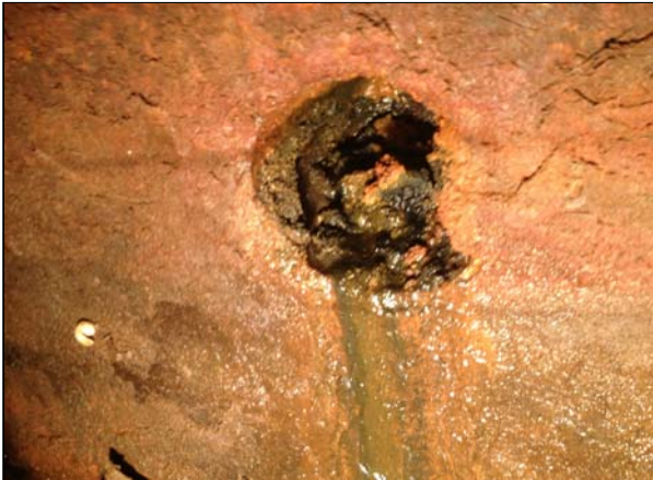
Photo 3: One of the 8-inch toe drains where sediment was sampled. 9/28/15
