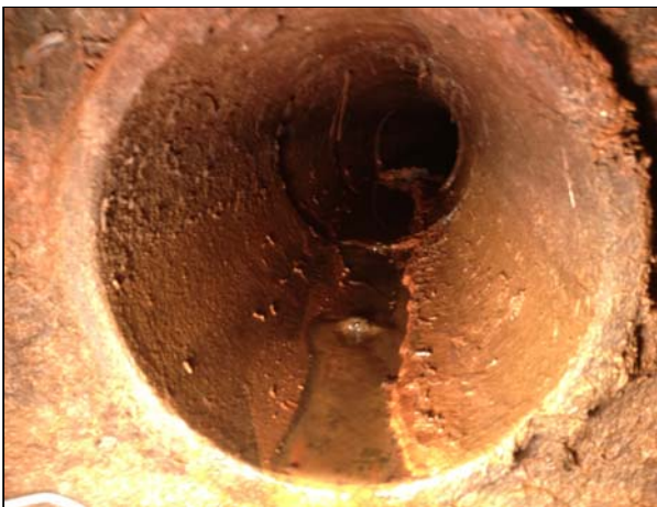
Photo 5: 12-inch collector drain coming into the Flood Gate Chamber from the east. 9/28/15
