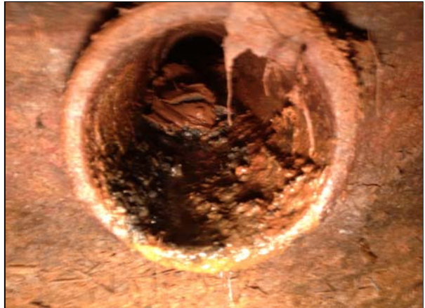
Photo 4: Other of the 8-inch toe drains where sediment was sampled. 9/28/15
