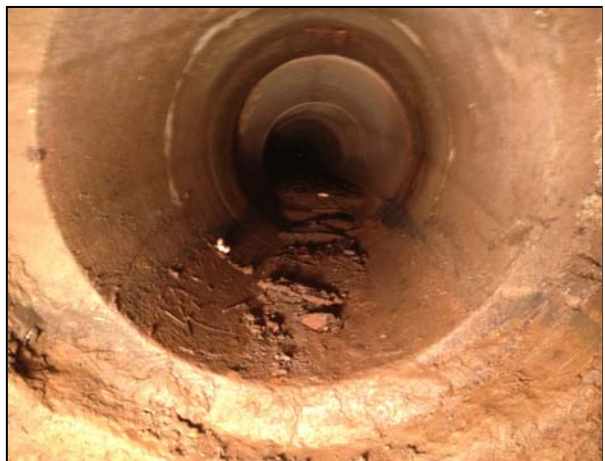
Photo 6: 24-inch collector drain going west toward MH4, MH5, MH6, and tailrace #2 at the Ames building. 9/28/15
