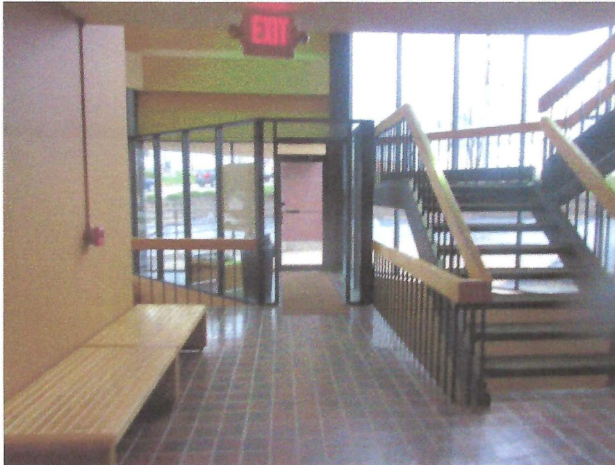
Interior view of building entry looking to subject unit
