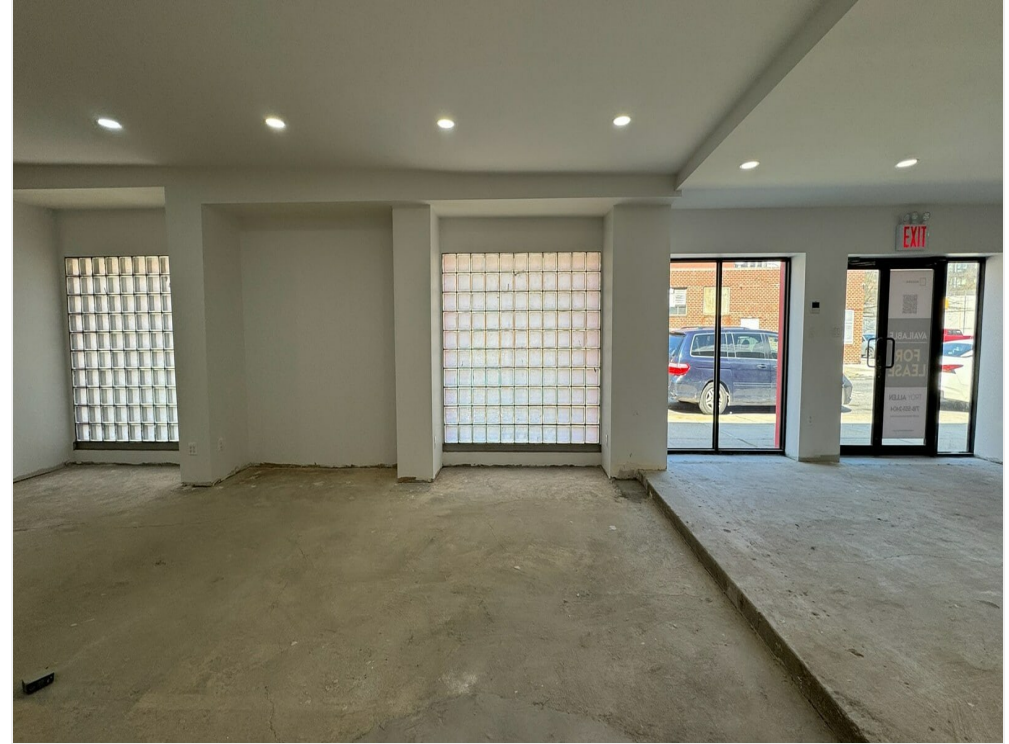
Main Building North Wall
