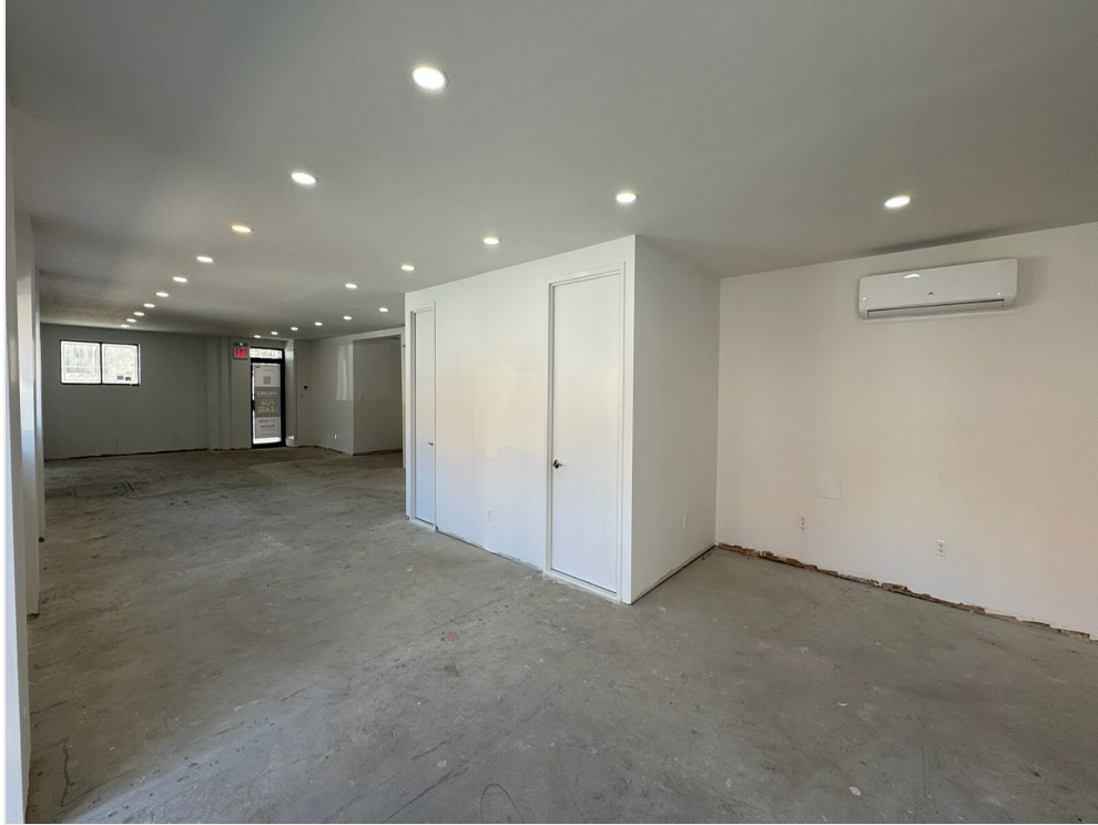
Main Building South Wall
