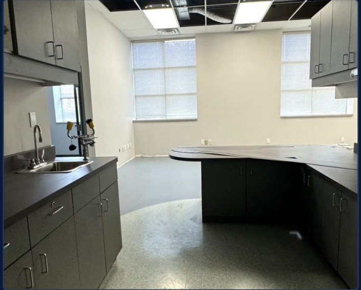
CLINICAL FIT-OUT IN PLACE · CASEWORK & SERVICES
