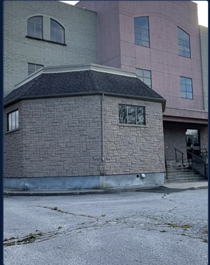
REAR / CORNER · PARKING & SERVICE ACCESS
