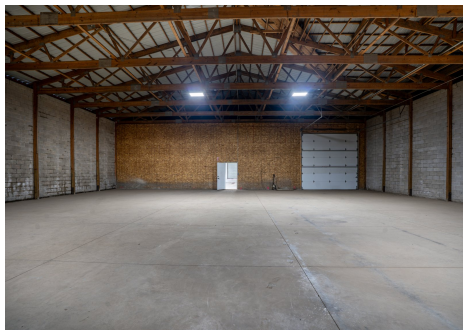
Clear-span, column-free interior
