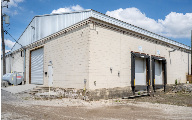
Unit B exterior — masonry warehouse with two dock-high doors (Dock 1 & Dock 2) and ground-level drive-in.
