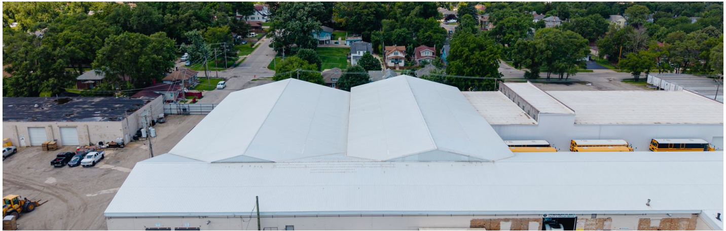
Aerial of the 807 Fourth Avenue industrial complex — Joliet, Will County, Illinois.
