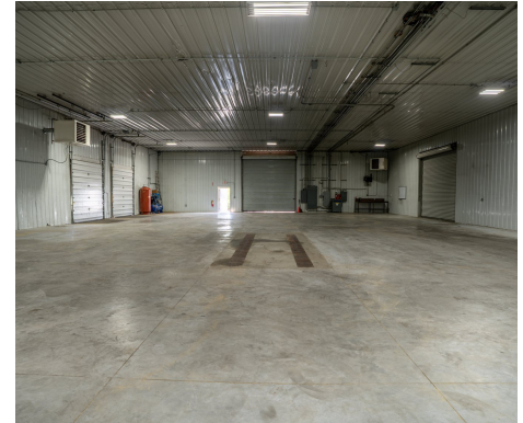
Clear-span finished warehouse
