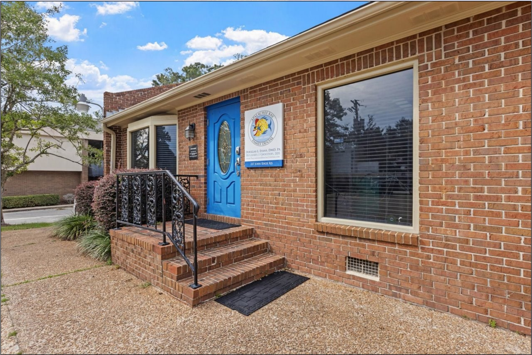
Front Entrance Exterior 237 John Knox
