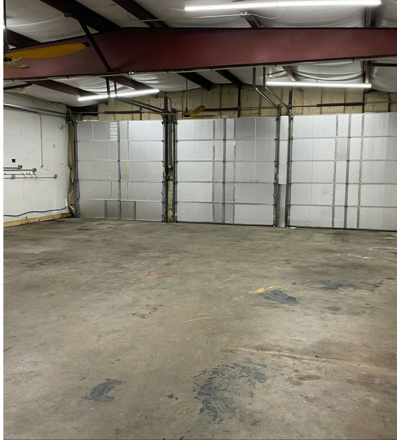
Shop with 3 Drive-In Doors
