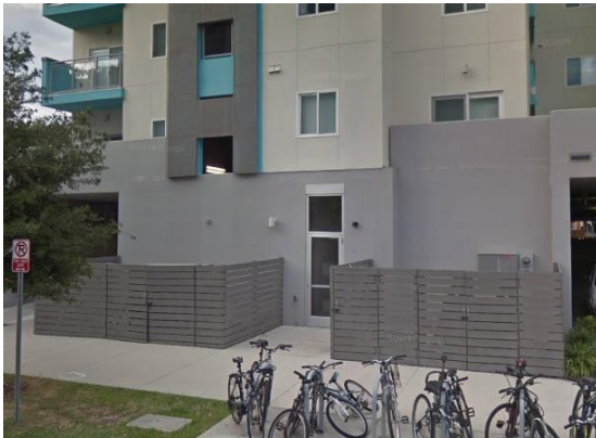
Allowed (utilities screened by fence)
