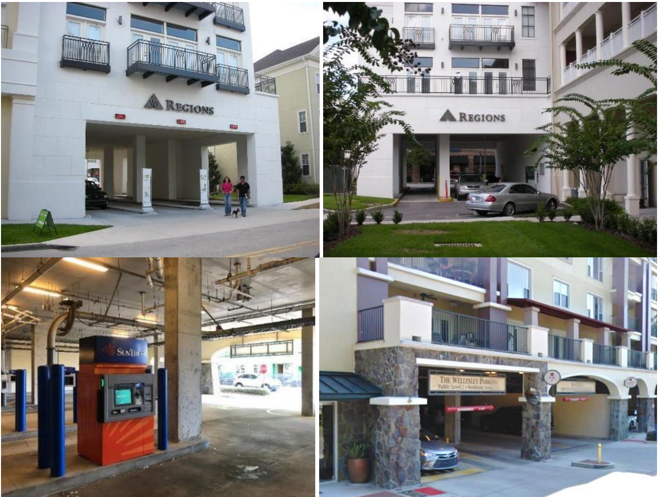
Figure 5 - 36: Interior Drive-Through Facilities
