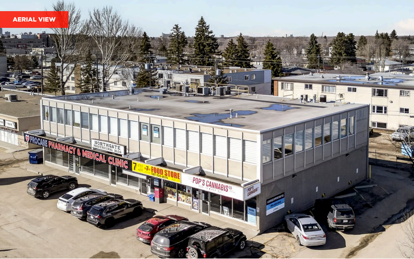
North elevation with full retail signage band and surface parking field along 97 Street NW
