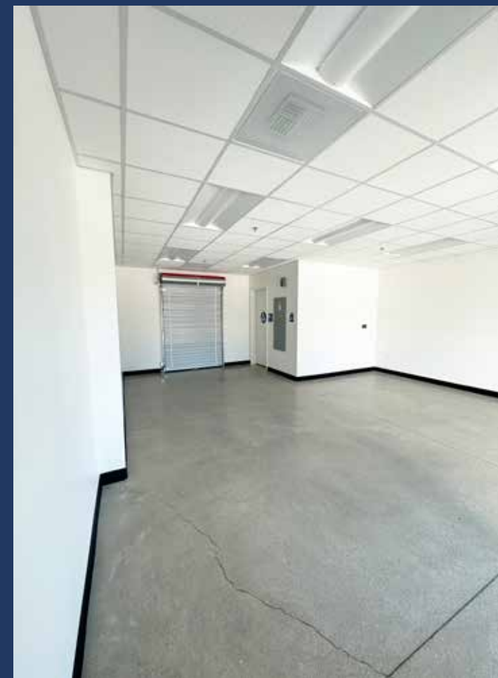
Roll up door, polished concrete flooring & restroom
