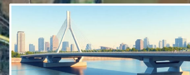
NEW I-55 BRIDGE
