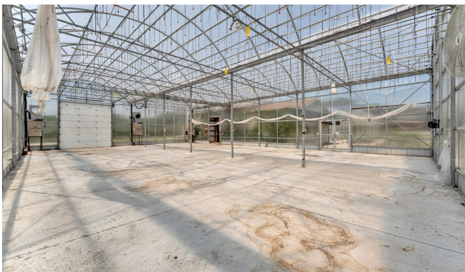
OPEN PRODUCTION AREA WITH CONCRETE FLOORING AND LOADING ACCESS
