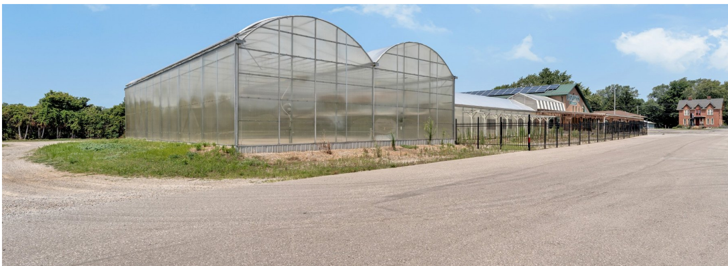
MULTIPLE GREENHOUSE STRUCTURES INTEGRATED WITH THE COMMERCIAL COMPLEX
