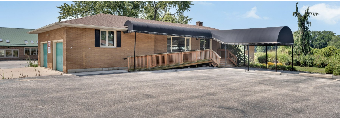
ACCESSIBLE COMMERCIAL BUILDING WITH PAVED ON-SITE PARKING
