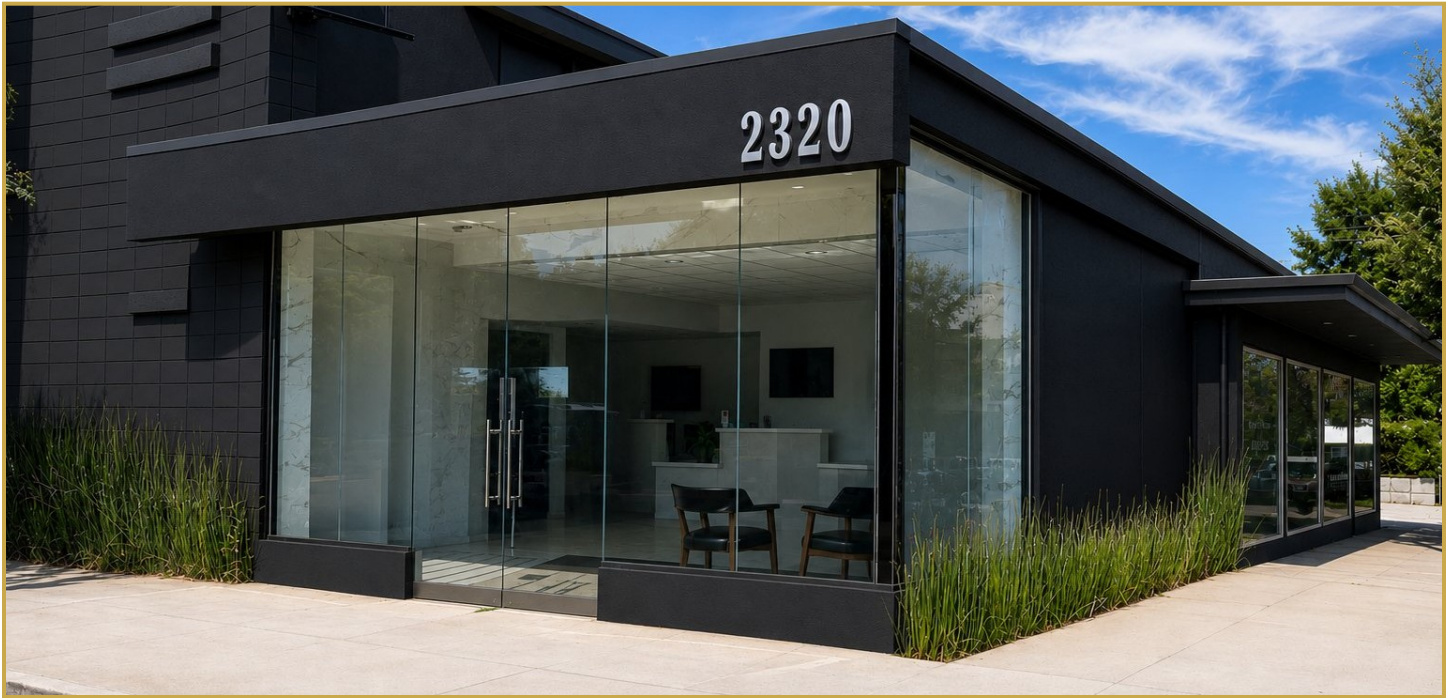
Building Exterior — 2320 S Robertson Blvd, Los Angeles, CA 90034
