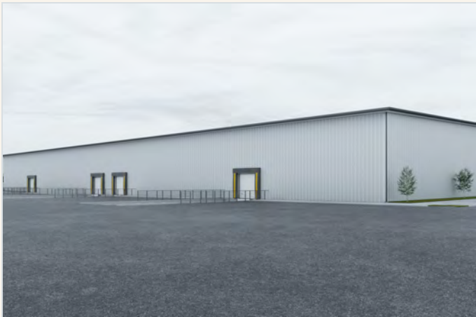
DOCK-HIGH LOADING & TRUCK COURT
