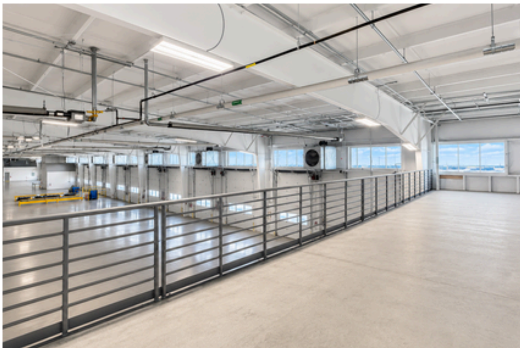
Mezzanine | Overlooks full warehouse floor
