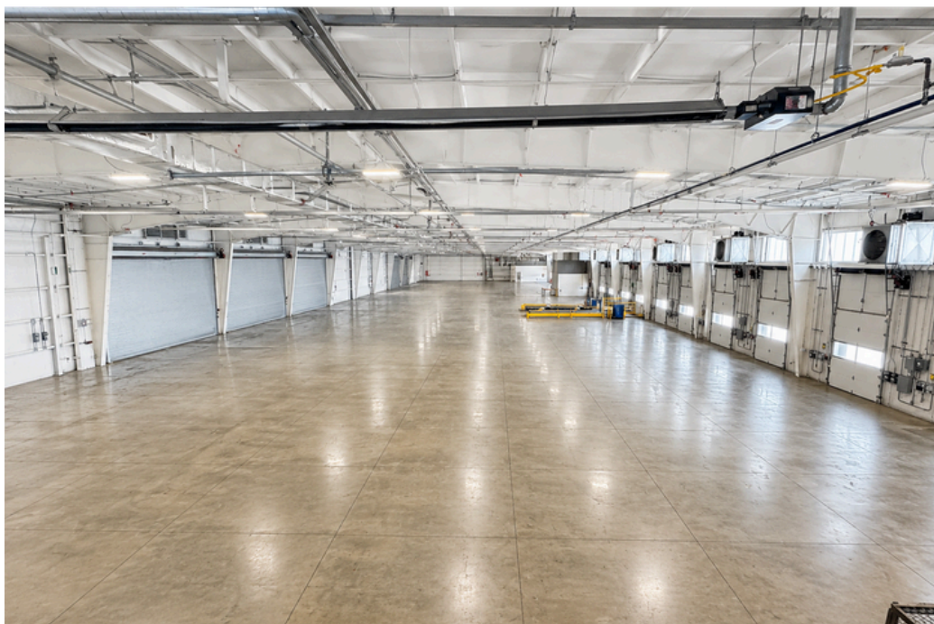
Warehouse Interior | Clear-span floor, add ceiling height here ceilings
