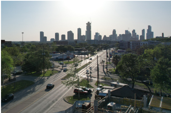
View from the 4th floor roof deck
