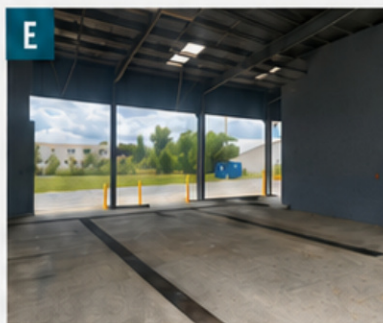
Warehouse #2 Drive-Through Interior
