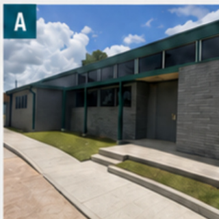
Office Exterior / Front Entrance
