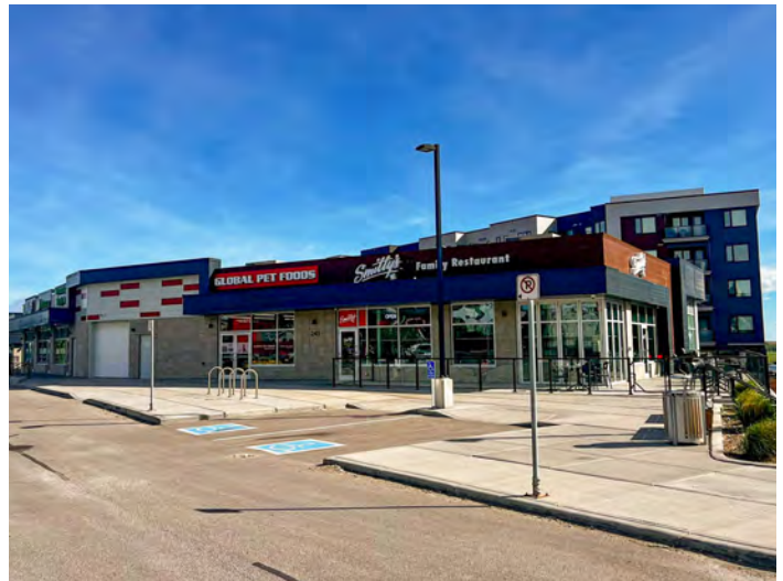
Building K - Upper Level - (Leased)
