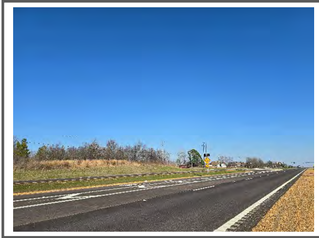
Goodmand Road site view and eastbound approach
