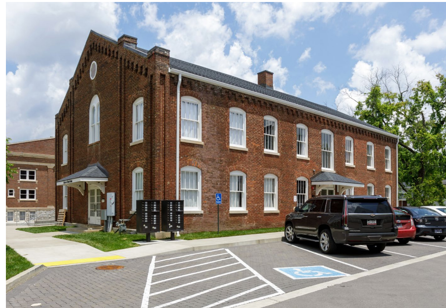
BUILDING D / 6,443 SF
