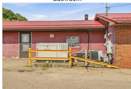
Side of Structure
