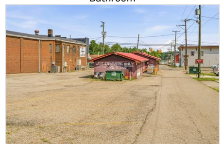
Back of Structure
