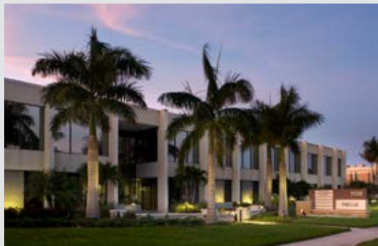
Building lighting & monument signage
