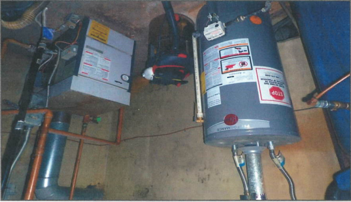
Subject Improvement – Interior View – Basement
