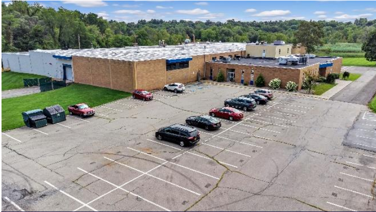
Exterior from West
