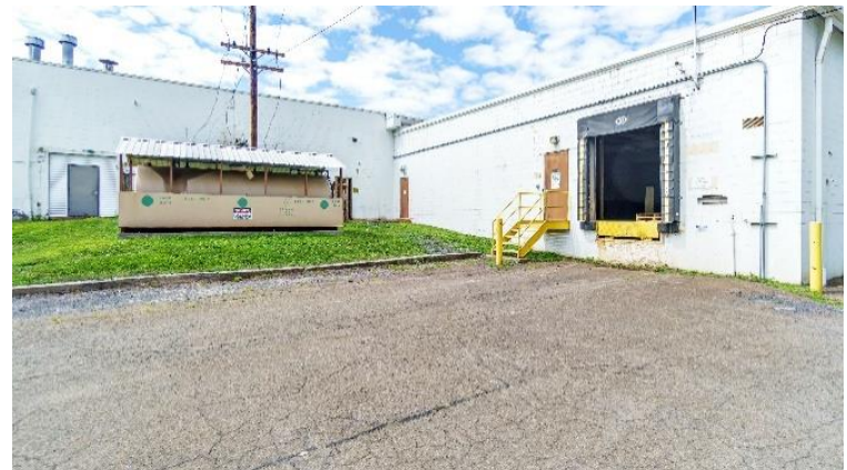
Loading Area - North Industrial Section
