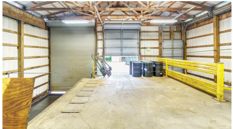
Loading Area – North wall of Main Section
