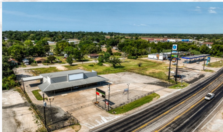
DIRECT HIGHWAY FRONTAGE
