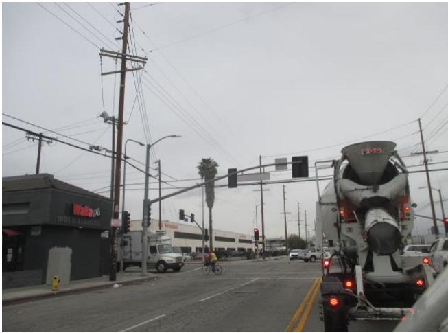
View north on Alameda St – subject on left
