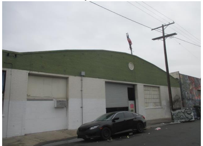
Subject industrial building on McGary Street
